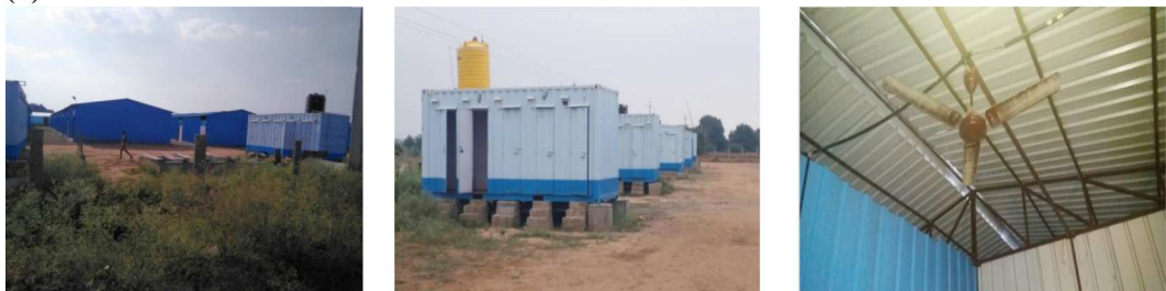
Fig. 3. Conditions of the labour dwellings: (A) Before intervention, and (B) After intervention, during a malaria outbreak in solar power project, Tumakuru, Karnataka.
